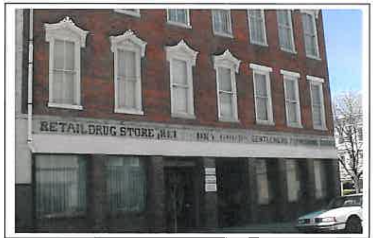
Historically, signs were often located in the storefront cornice area, as seen on this Pearl Street building.
