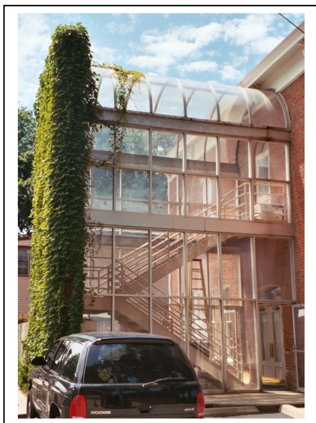
This addition is clearly distinguishable as new, yet fits in with the historic German-American Academy.
