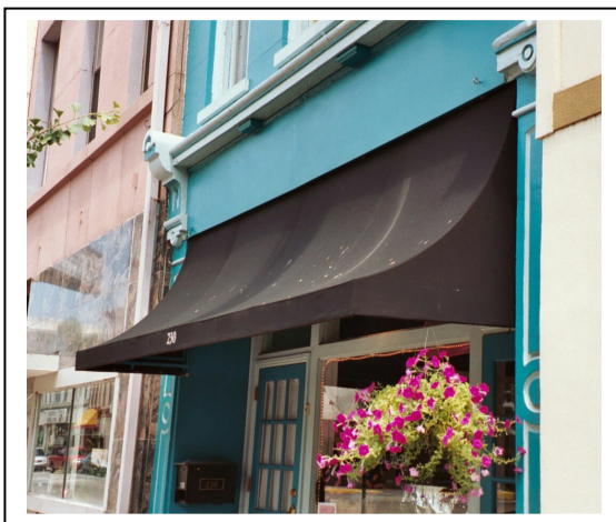
Concave awning on Pearl Street.
