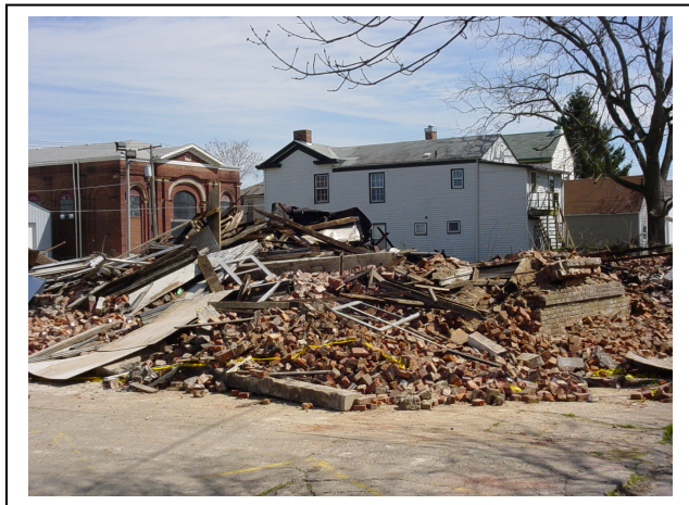
Deferred maintenance led to the collapse of Maennechor Halle on East Spring Street in February 2003.
