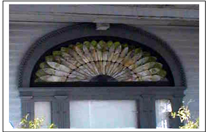
The stained glass fanlight is a character-defining feature of this West Market Street home.
