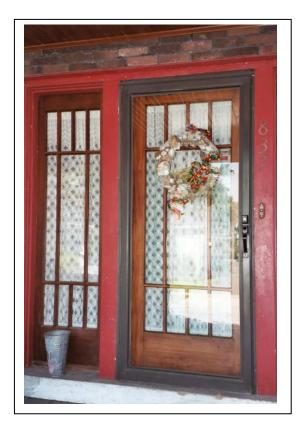
This full glass storm door allows a good view of the Craftsman-style door behind it while also increasing energy efficiency.
