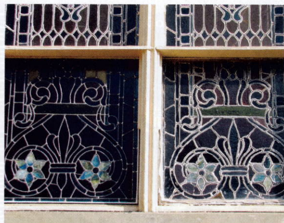
LEFT: Notice the bulging section, and missing and cracked glass in this 1920s staircase window. RIGHT: The bottom left side has been restored on this pair of 1920s panels. (Right side is before restoration.)
