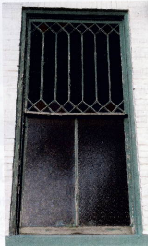
LEFT: Deferred maintenance and inadequate past installation results in this condition. RIGHT: Evidence of deteriorated wood and window sash.
