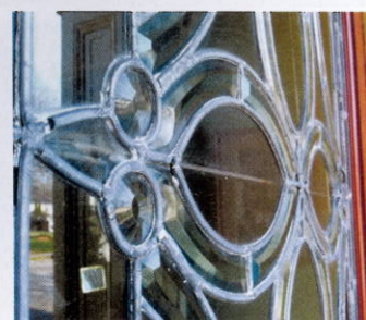
FAR LEFT: The upper window needs glass replacement. LEFT TOP: A transom damaged by high winds is in need of glass replacement. LEFT BOTTOM: This panel suffers from brittle waterproofing putty as well as buckling. MIDDLE: Notice the broken solder joints and bulging in this zinc-channel door panel; it will need to be removed to repair it. ABOVE: This leaded door panel suffers from broken solder joints and loose waterproofing putty.
