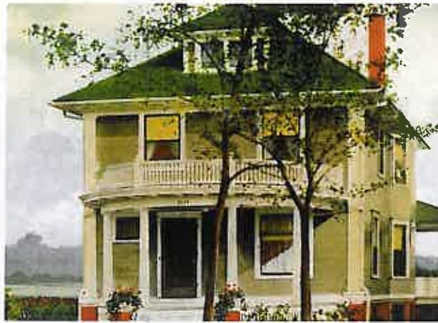
Cream trim, lighter than the olive-green body color, enhances the Colonial Revival spirit of this American Foursquare, drawing attention to the columns, corner pilasters, and balustrades.
